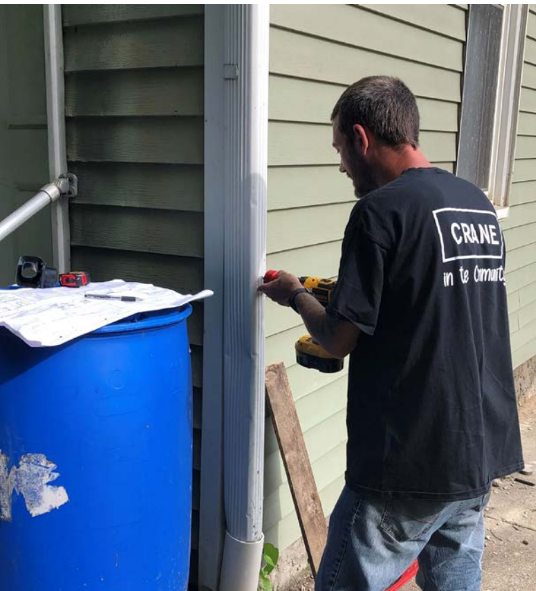
Crane ChemPharma & Energy associate in Cincinnati, OH helps to install a downspout diverter to feed into a wooden planter box, recycling rainwater for use in the garden. This site has done multiple projects in the community with Working In Neighborhoods throughout the year.
